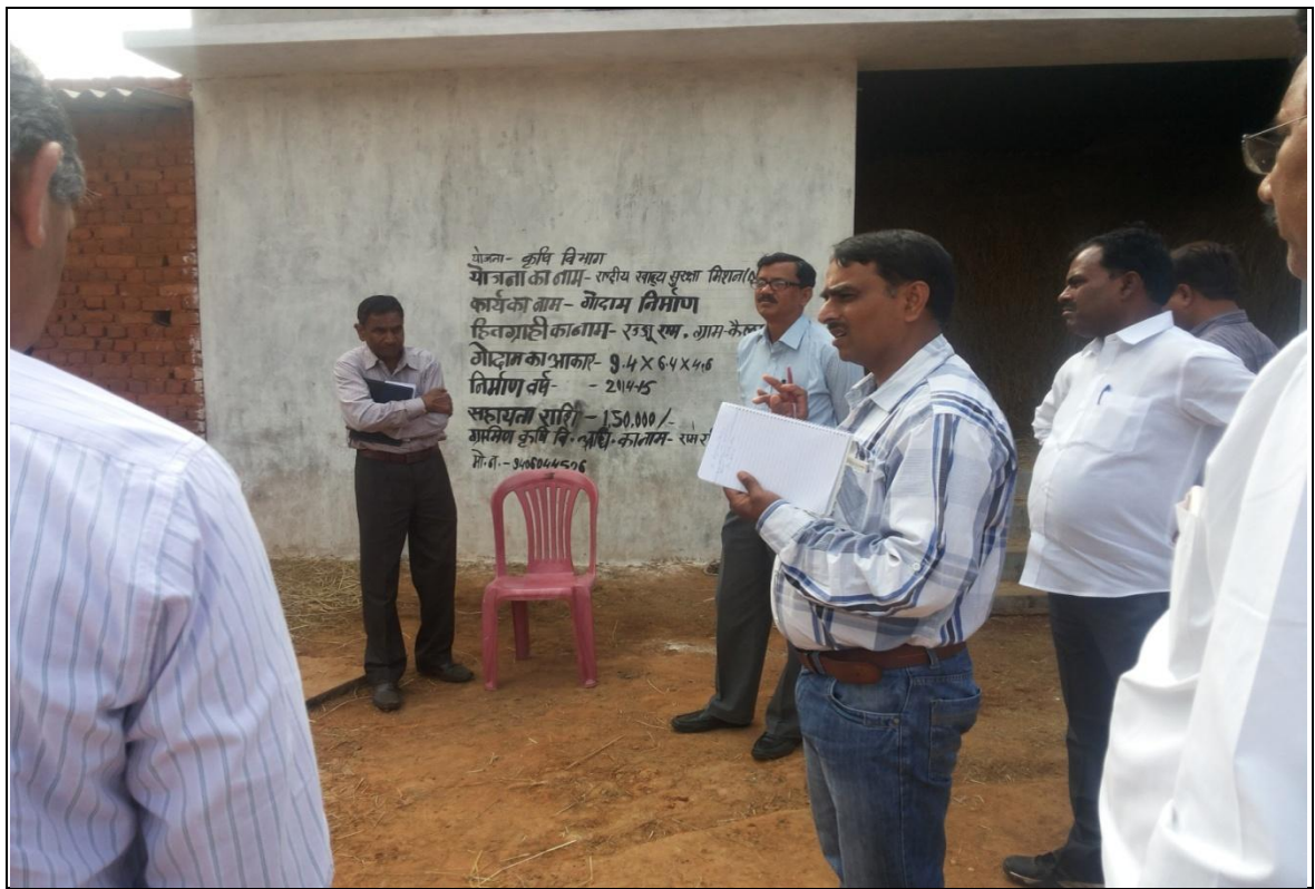
Local Initiatives: Godown constructed under NFSM- Pulses, 2015-16 District-Surajpur, Block-Surajpur, Village- Kailashpuri,
